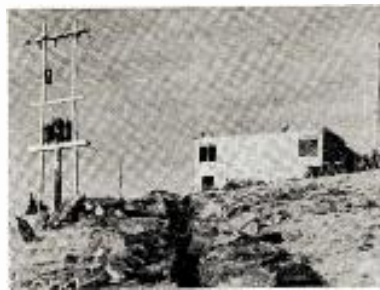
KXLY-TV transmitter building now under construction. ➤
